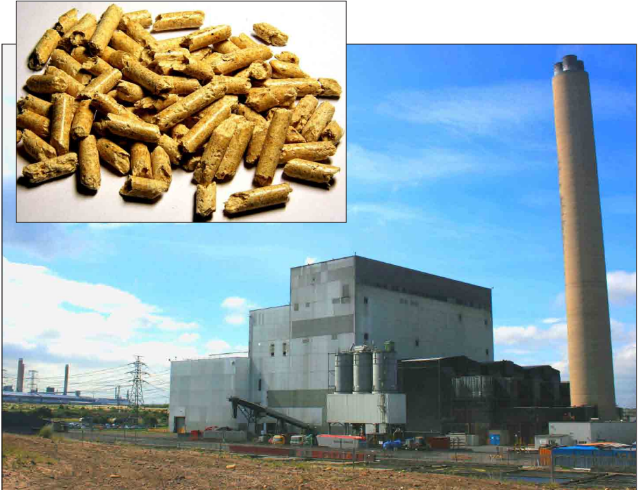
Lynemouth power station, England; formerly coal fueled, then fueled with wood pellets. Credit: Wikimedia, D. Kuru.
