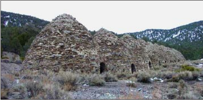
Ten stone kilns built in 1877, each 7.5m tall, formerly to supply charcoal for metal smelters in Panamint Valley, California. Pinyon pine and juniper woodlands on surrounding hills supplied the wood. Credit: Wikimedia.
